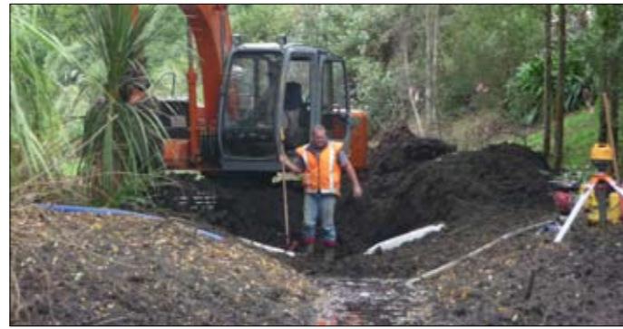
Dormer Construction creating the swale, April 2009.
